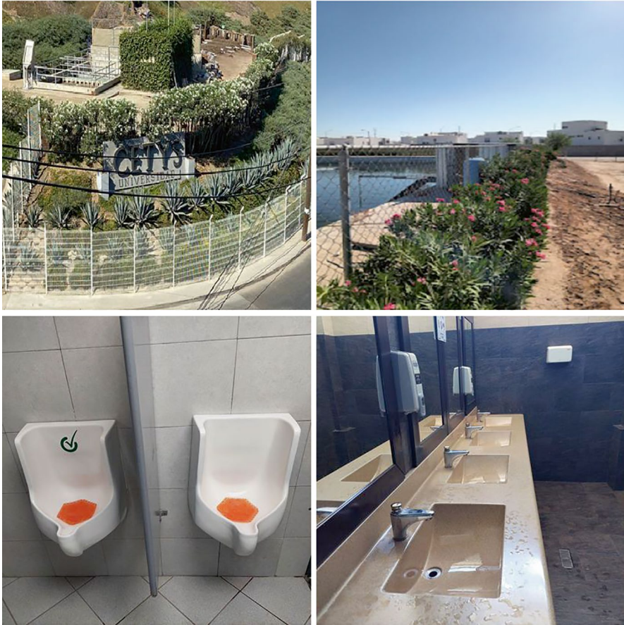
Fig. 2 Examples of wastewater treatment plants (upper) and water efficient usage appliances (bottom)
